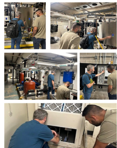
Figure 12: HVAC controls training for trades team
