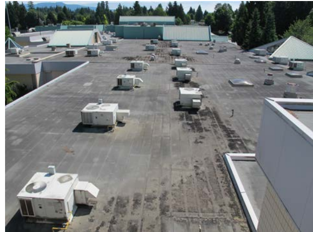
Figure 4 – Sample RTU's to be replaced with Air Source Heat Pumps
