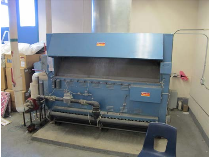
Figure 1- Domestic Hot Water Boiler
