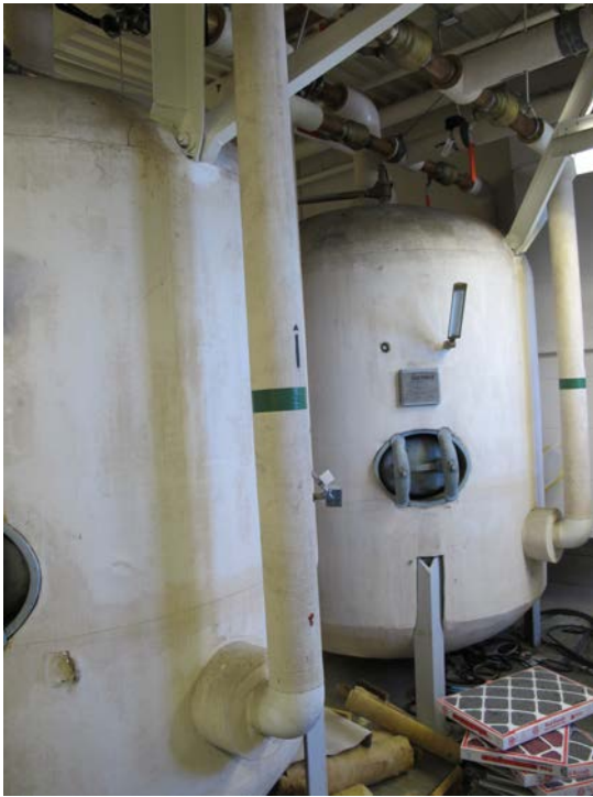
Figure 3 – Domestic Hot Water Storage Tanks
