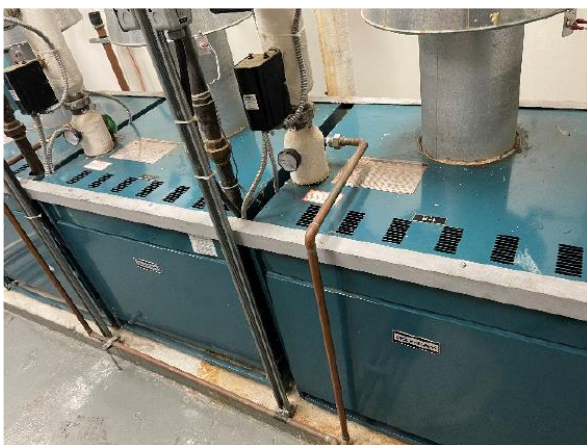
Old Atmospheric Boilers
