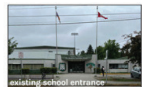
existing school entrance
